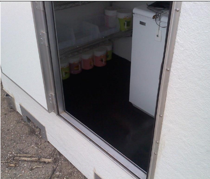
Rubber mat flooring easily removed and cleaned
