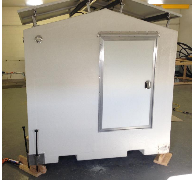
Simple stake system to secure in high winds
