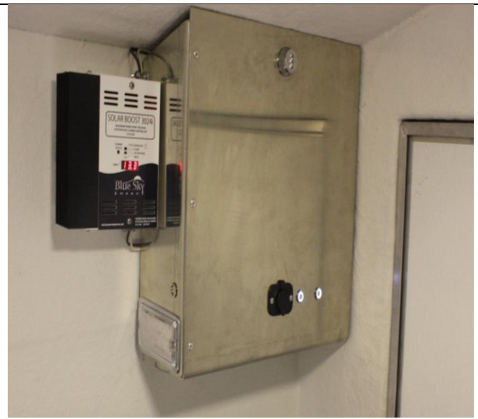
Battery and Control box with USB port for charging laptops and phones for medical uses
